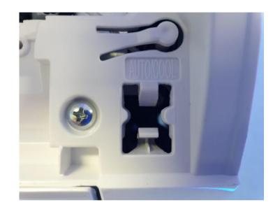
Lift up the fascia to reveal the Forced cooling button on the bottom right of the unit, below the wiring terminals
