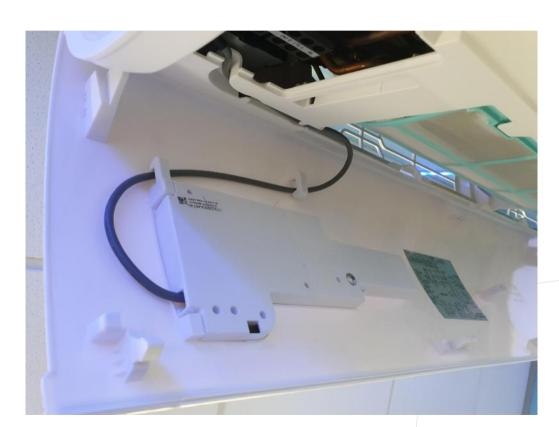
The connections for both the wifi adapter and a hard wired controller are on the display board
